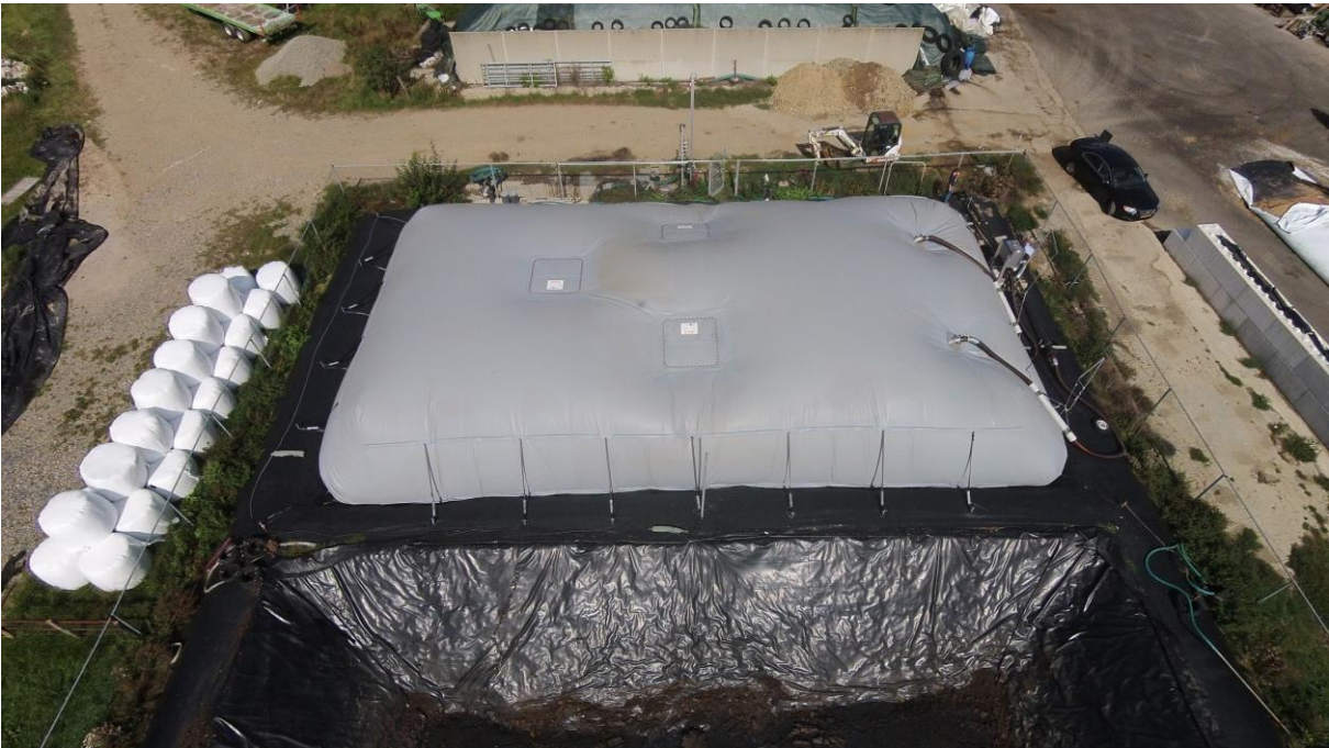
Figure 3 - Installed Biogas lagoon (Nidrum, Belgium)
